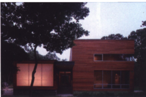
The garage, visible from the street, is made attractive with acrylic panels from CYRO Industries. “When the garage is illuminated at night, it glows nicely,” says architect Carol DiCicco Vinci.
